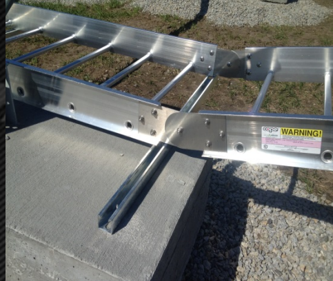
Cable trays mounted on ballast blocks
