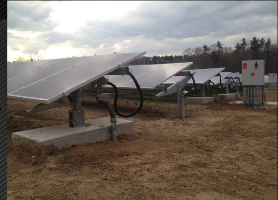
Hybrid Ballast with Post Driven System
